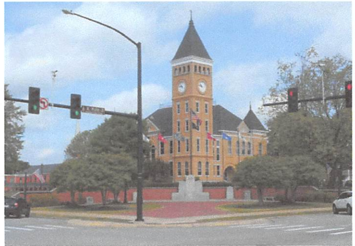
Benton's Courthouse square contributes to a sense of place downtown.
