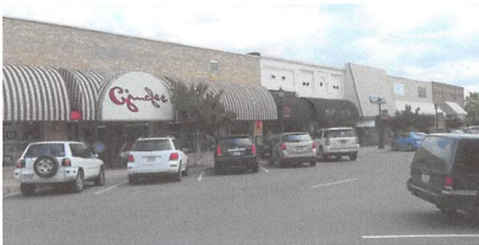
Downtown retail combines variety and walkability, while costing taxpayers less to develop and maintain.
